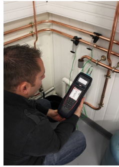
DHW network temperature
